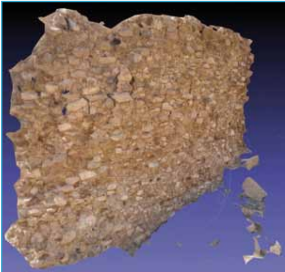
Fig. 8. 3D model of the north wall of the Paikuli monument, acquired through the Menci ZScan system
