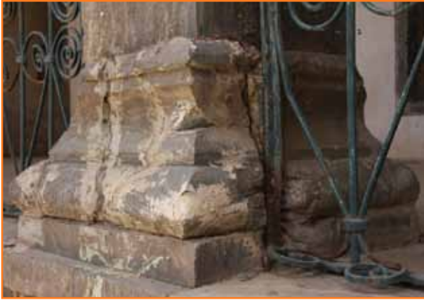
Fig. 2. Base of the loggia pillar
